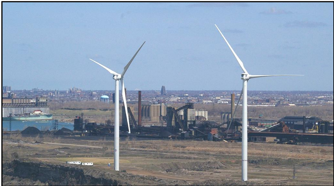
Steel Winds Urban Wind Farm, Buffalo, New York
