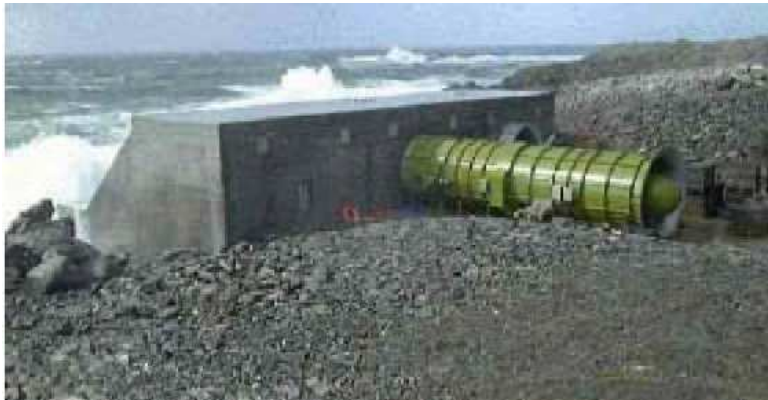
Figure 7: "Limpet" OWC at Isle of Islay, Scotland
