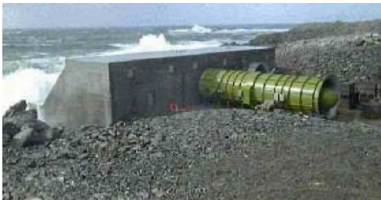
Figure 7: "Limpet" OWC at Isle of Islay, Scotland
